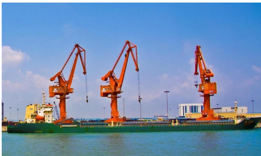
Photo plate 3-3: Container Quay Crane
