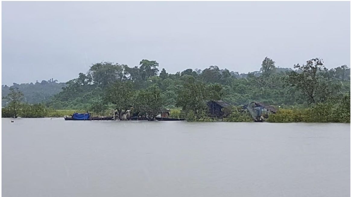
Photo plate 4-3: Shoreline along Made Island Terminal quay line
